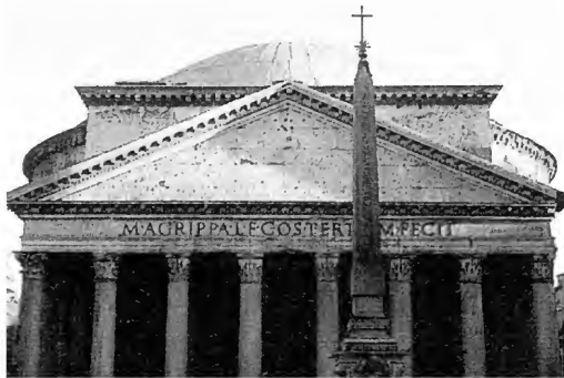
Fig. 7.80. A XVIII century obelisk in front of the façade of the "ancient" Pantheon allegedly built in the II century A.D. One can clearly see that the XVIII century obelisk resembles other "ancient" Egyptian obelisks in style. Apparently, the recent XV-XVII century tradition of building similar Christian obelisks still existed in the XVIII century. Taken from [726], page 61.
