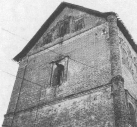
Fig. 14.230. Old building at the New Simonov Monastery in Moscow. The construction is most likely to have been an old Russian church with a gable roof, later converted for drying corn. Photograph taken in 2000.
