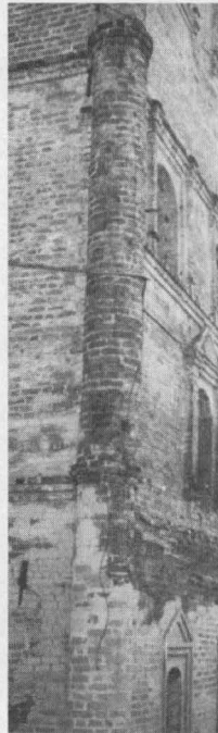
Fig. 14.231. Old building at the New Simonov Monastery in Moscow. The tower, or column, integrated into the wall of the building and typical for Western European cathedrals, is visible perfectly well. Photograph taken in 2000.
