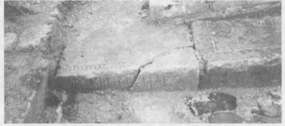
Fig. 14.38. Headstones of white stone with triangular crosses immured in the foundation of a XVII century church. One of them is marked "7 February 7191". The dating converts into the modern chronological system as 1683 A. D. Louzhetskiy Monastery, Mozhaysk. Photograph taken in 2000.
