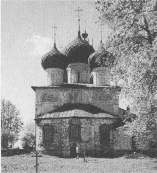
Fig. 14.218. A typical Russian church of the XVII century. This is the Nikolskaya Church of the Nikolo-Ouleymenskiy Monastery near Ouglich. We see the eastern wall of the church. It is presumed that most Russian churches of the XII-XVI century had looked like this.
