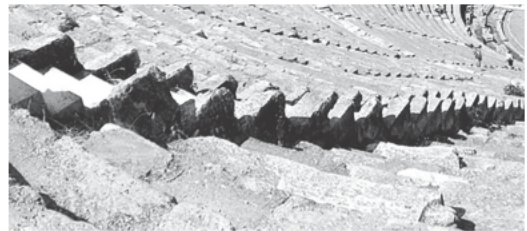
Fig. 19.88. Close-in of the fragment with the eroded stairs of the Ephesus amphitheatre. We can clearly see the inclusions of gravel and pebbles in the “ancient” concrete. Taken from [1259], pages 88-89.
