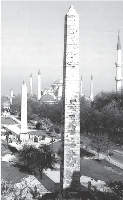
Fig. 19.65-66. Obelisk (column) of Constantine VII Porphyrogenitus allegedly dating from 940 A. D. It stands at the Istanbul Hippodrome. The construction is made of stone blocks covered in a layer of cement. The cement and the exterior have peeled off over the years.
