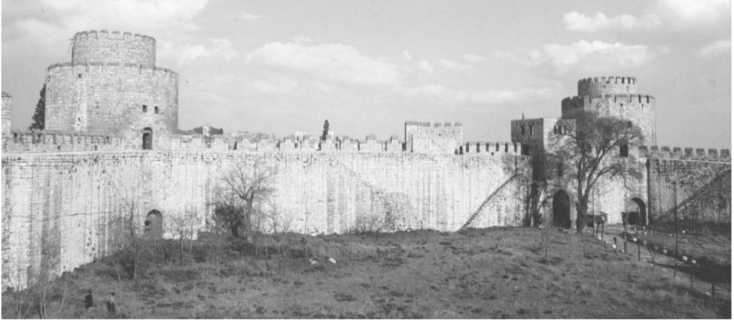
Fig. 8.5. Partially restored part of Constantinople wall. Taken from [1464], page 80.
