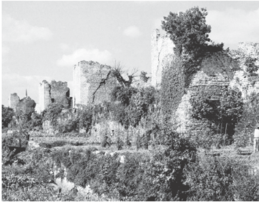
Fig. 8.4. Seriously damaged part of Constantinople wall. Taken from [1464], page 78.
